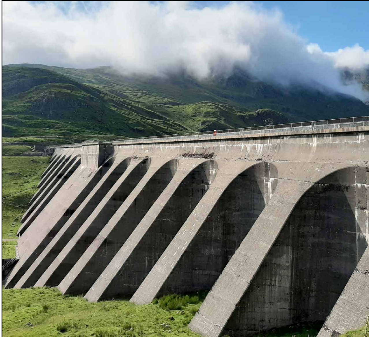
The 316-metre long buttress dam at Cruachan Reservoir is the obvious landmark in the upland areas of the survey site
